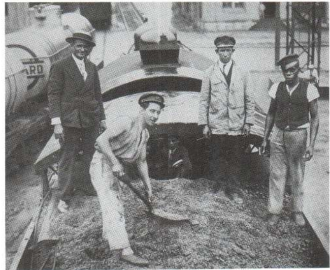
Mixing coffee into tar to be used in building new roads and highways.
